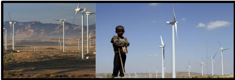
Fig. 3.9 Ashegoda wind farm near Mekelle
